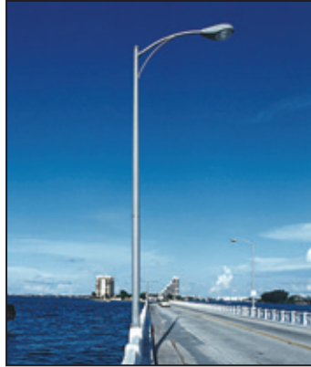
Venetian Causeway Miami, FL Installed Circa 1951
