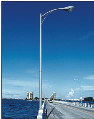
Venetian Causeway Miami, FL Installed Circa 1951
