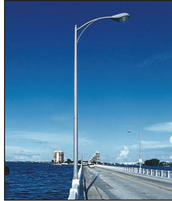
Venetian Causeway Miami, FL Installed Circa 1951
